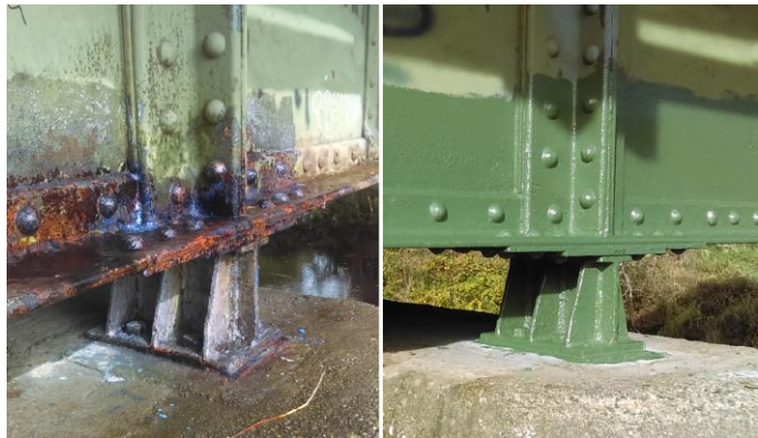
FHWA Bridge Preservation Guide (2018)
