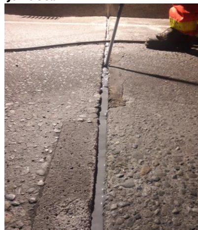
FHWA Bridge Preservation Guide (2018)
