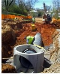
Public Works in Action: Replacing a stormwater pipe
